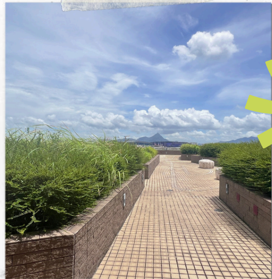
Figure 5-10: A green roof to reduce the temperature on the top floor
