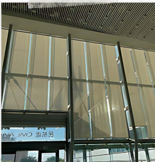
Figure 5-8: Motorised blinds in atrium
