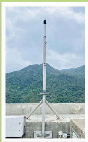
Figure 2-4: Outdoor noise monitoring terminal
