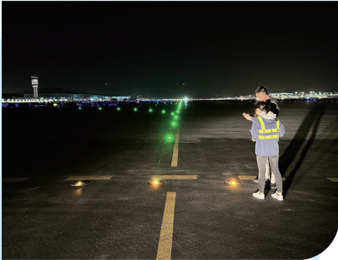
APSD colleagues conducted compliance check on airfield ground lighting.
